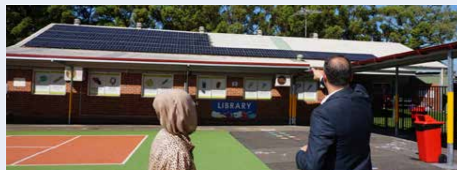
Greenacre PS new Solar Panel thanks to Community Building Partnership Grants
